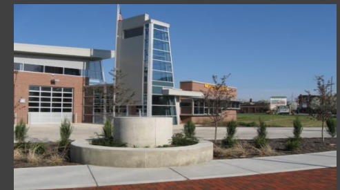
City of Cincinnati, Fire Station #51
