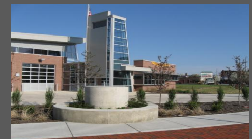
City of Cincinnati, Fire Station #51
