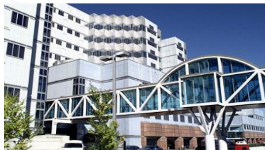
Portland VA Medical Center, Portland, OR
